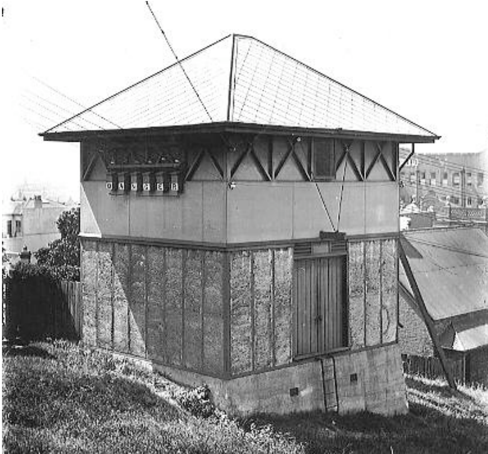
Figure 9.42. Electrical Substation, King Street, Newcastle. Source. Hunter Photo Bank.
