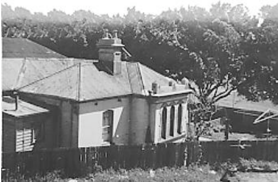
Figure 7.14. Signalman's Cottage at the junction of the A A Company and Merewether Mine rail lines near what is now Civic Park. Source. Hunter Photo Bank.
