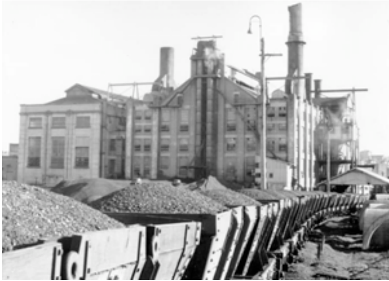
Figure 9.41. The Zaara Street Power Station, Newcastle, 1949. Source. Hunter Photo Bank.
