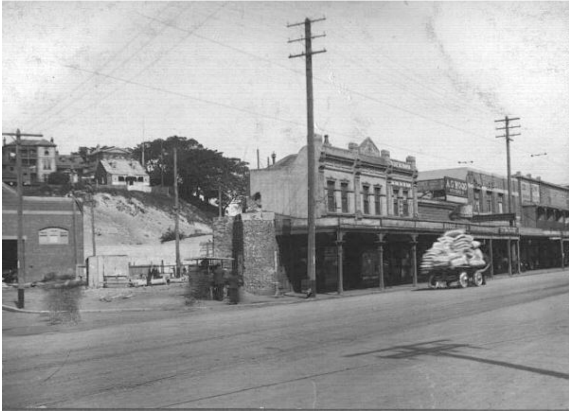
Figure 7.13. View of Hunter Street, showing the final stages of demolition of the Hunter Street bridge, 1920. Note the brick abutment adjacent to the shops on the right. Source. Hunter Photo Bank.
