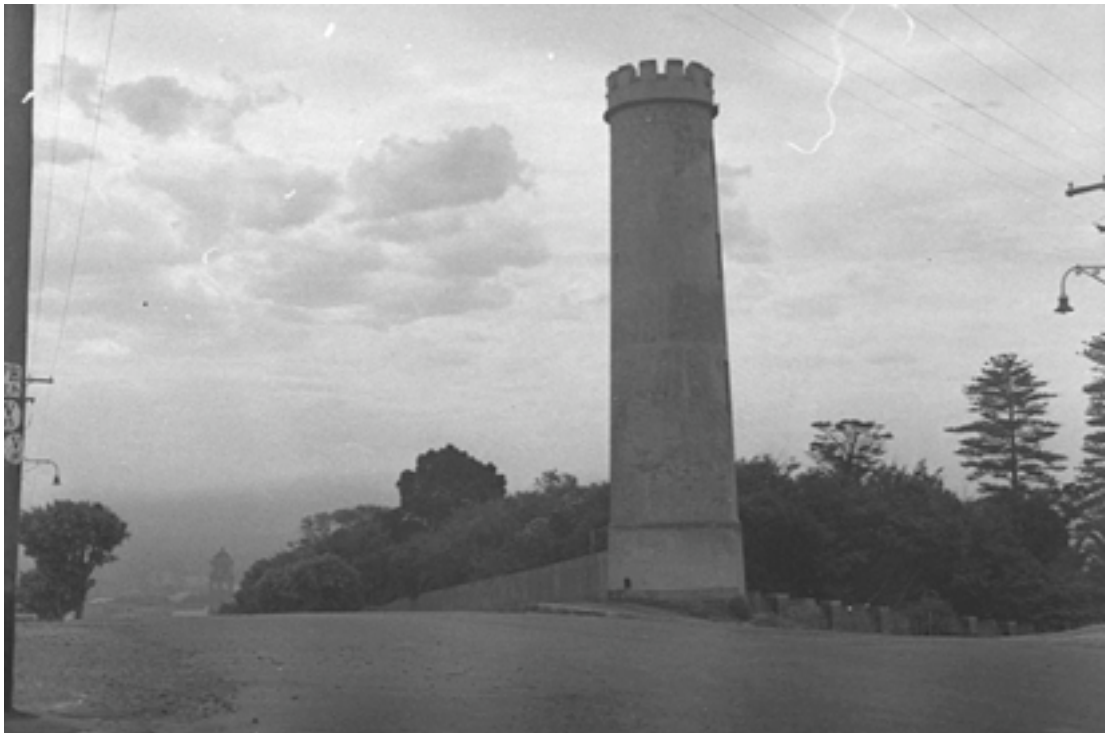
Figure 8.30. Navigational Beacon, Brown Street, Newcastle, 1953. The beacon was one of two erected in 1865. Source. State Library NSW. Digital Order No. hood_27224h
