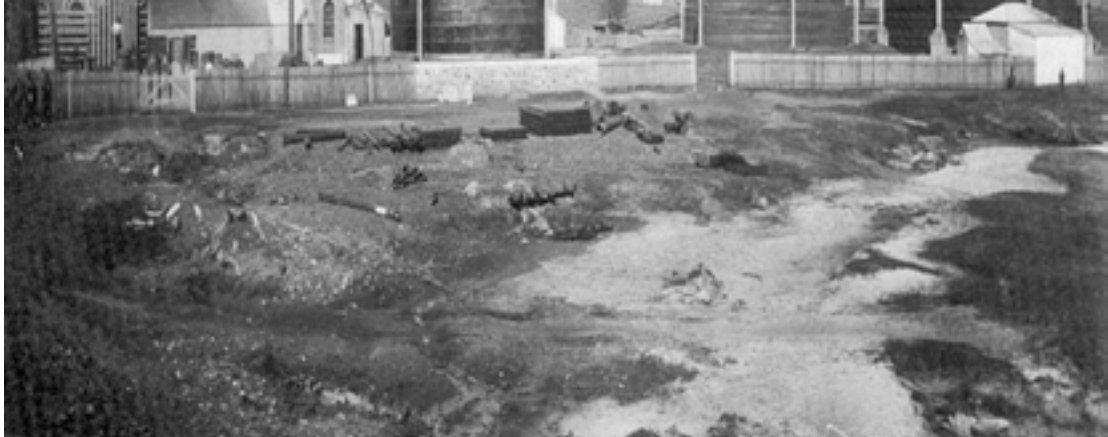
Figure 9.39. Gasworks, Parry Street, Newcastle, in c.1885. Source. State Records NSW. Digital Order No. bcp_05283.
