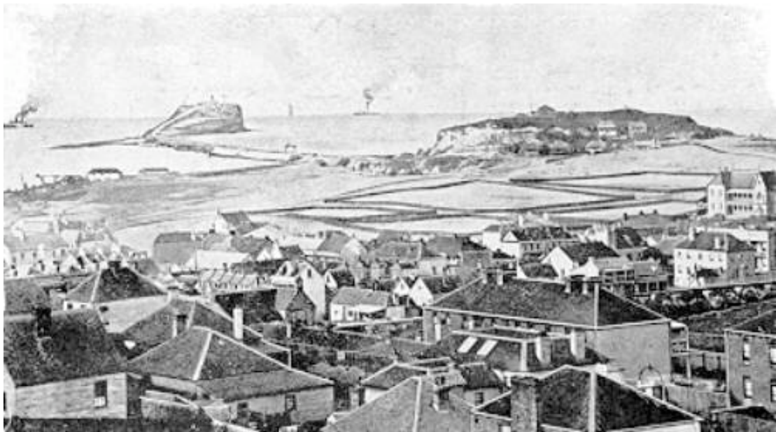
Figure 9.12. View of Newcastle and Nobbys Head c.1865. This view of Newcastle reveals the extent of development between 1850 and 1865. Note also that the Sandhills area in Newcastle East has been enclosed. On the flank of Flagstaff Hill are a number of buildings. Source. Hunter Photo Bank.
