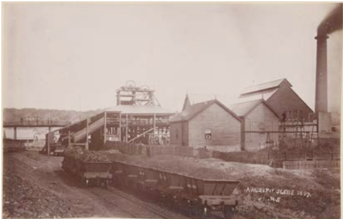
Figure 7.16. The AA Company's Glebe Colliery in 1887. Source. Hunter Photo Bank.
