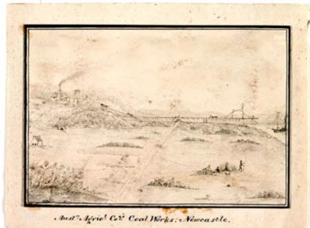
Figure 7.1. The "Austn Agricul Coy Coal Works, Newcastle", 1833. This picture shows the A Pit, opened in 1831, together with the inclined plane, the swing bridge over Hunter Street and the coal staithes of the AA Company, looking west. Source. State Library of NSW. Digital order No. a128615h
