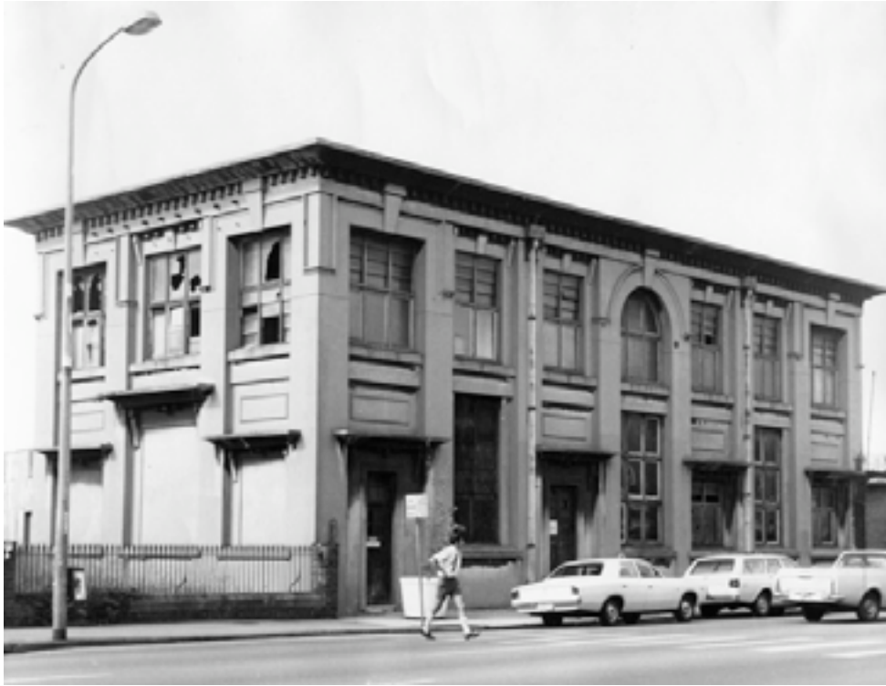
Figure 9.43. Electrical Substation, Hunter Street, Newcastle. Source. Hunter Photo Bank.
