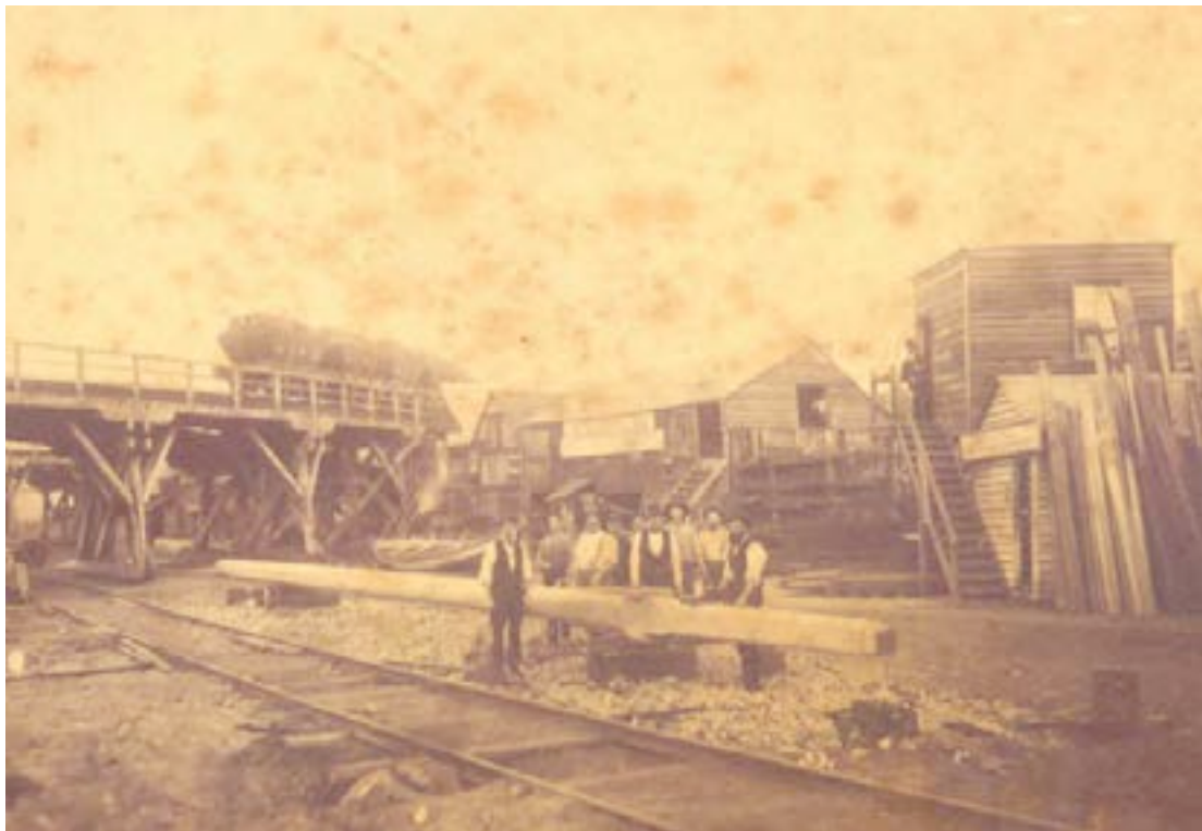
Figure 7.8. Wharf at Newcastle.
