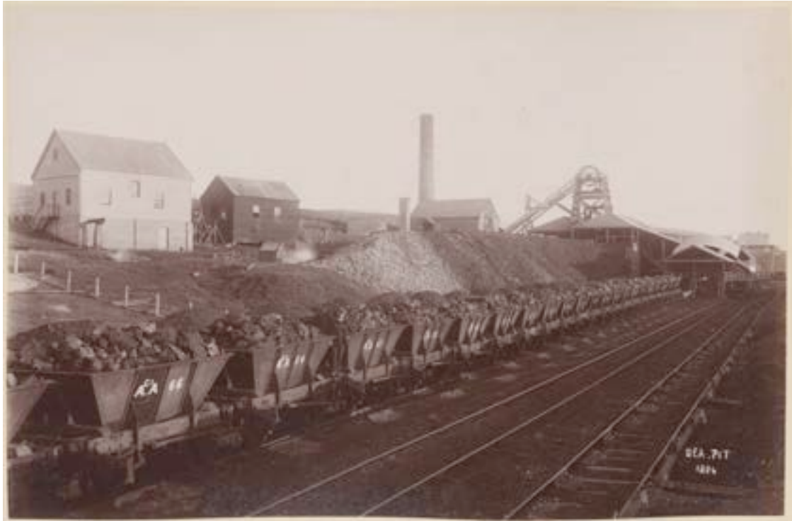
Figure 7.19. AA Company Sea Pit Colliery, near Darby Street, Cooks Hill, from the north. Source. State records NSW. Image No. 10036_a02700016.
