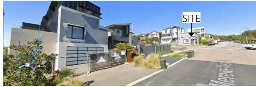
LOOKING STH TOWARDS SITE
