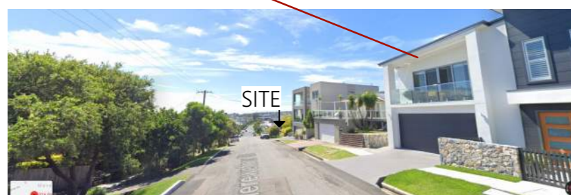
LOOKING NE TOWARDS SITE
