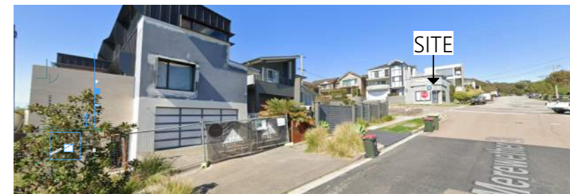
LOOKING STH TOWARDS SITE
