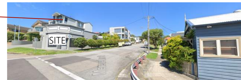
LOOKING STH TOWARDS SITE
