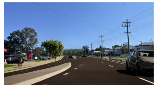
View facing east along Minmi Road
