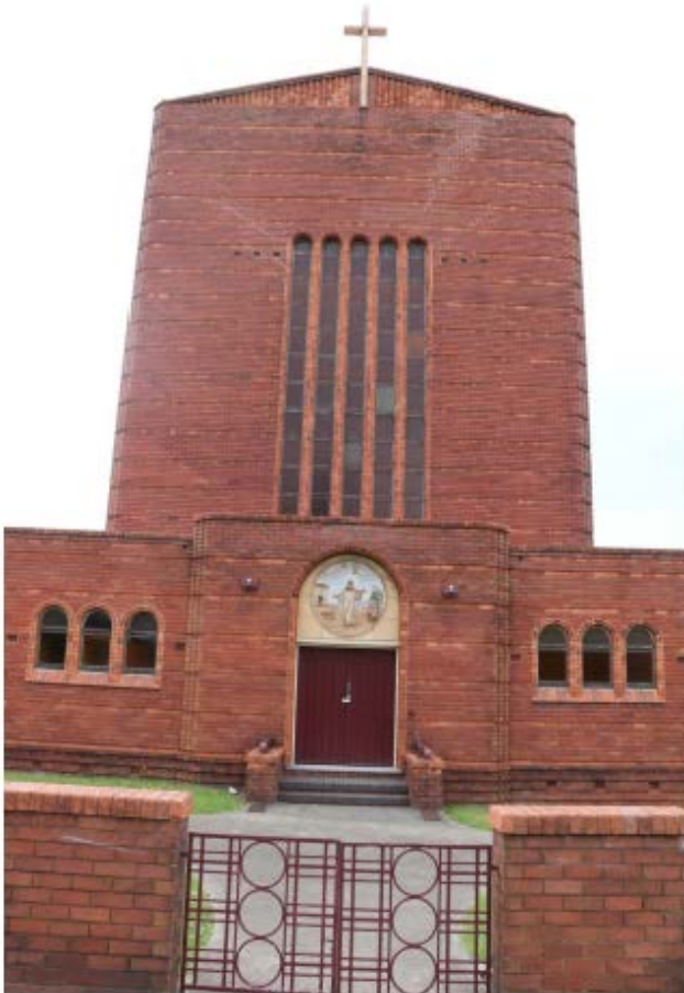
Photo 1: View of St Columban's from Church Street
