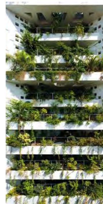
LANDSCAPED MASONRY PLANTERS
