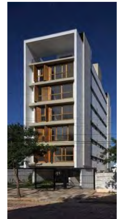
EXPRESSED CONCRETE SLAB & WALL EDGE
