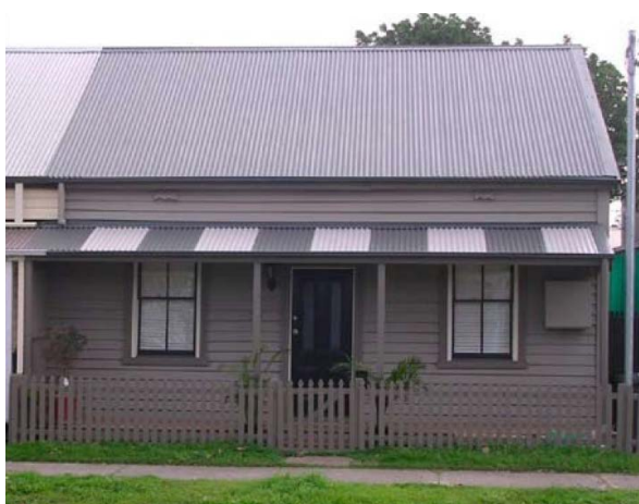
Figure 11: Example of an Early Victorian house, Coomes Consulting (2006)
