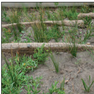
Slope stabilisation techniques
