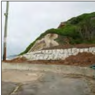
Headland with stabilised slope behind Baths Pavilion
