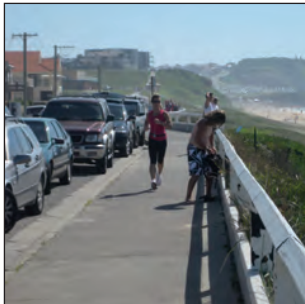
Existing footpath along John Parade
