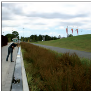
Swale, Armory Wharf
