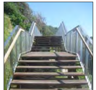
Timber stairs with open steel railing
