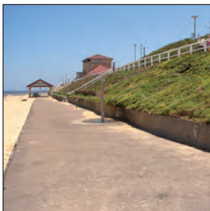
Sloped bank, retaining wall and promenade
