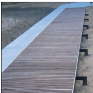
Timber walkway, Ballast Point
