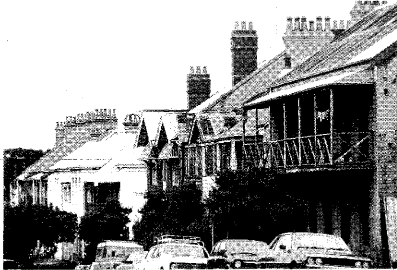
Chimney Pots. Townscape details. Church St.
