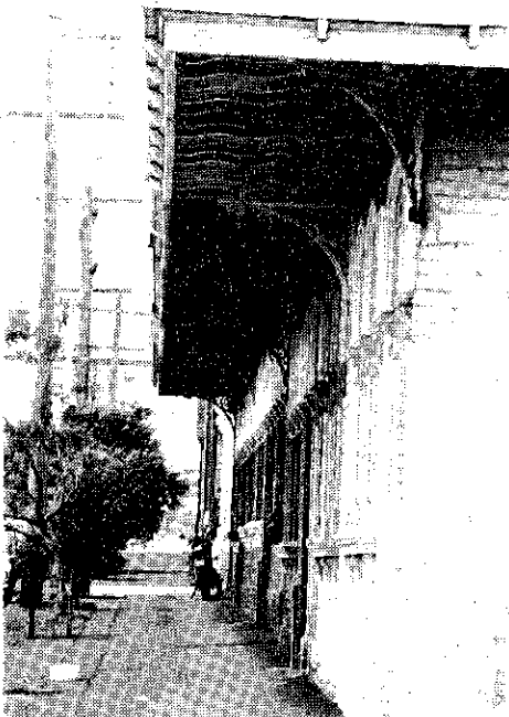
Cantilevered Balconies - Stevenson St Should be retained / reinstated. Note brackets + joint details.
