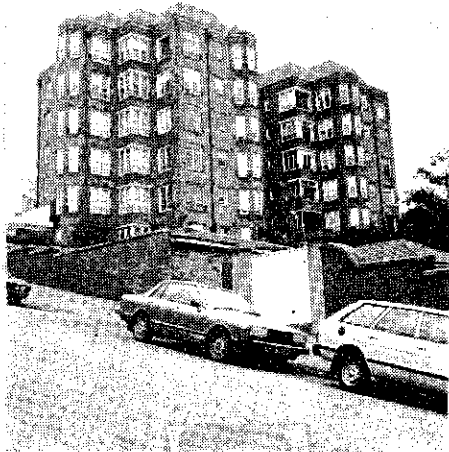
Segenhoe Apartments Arch: Emil Sodersten 1937. Unsympathetic facsimile tile roofing.
