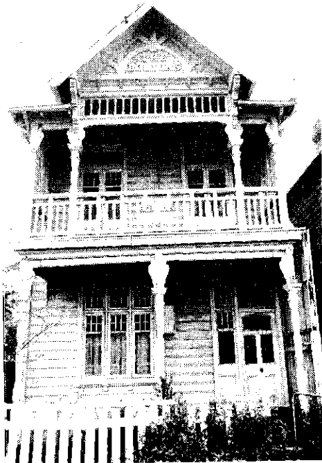
The Bolttons - Timber cladding and elaborate timber detailing.
