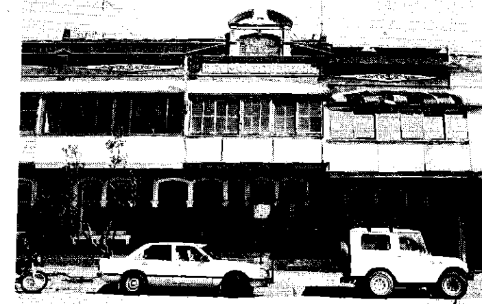
Stevenson Place - low quality balcony infill. Restoration should be encouraged.
