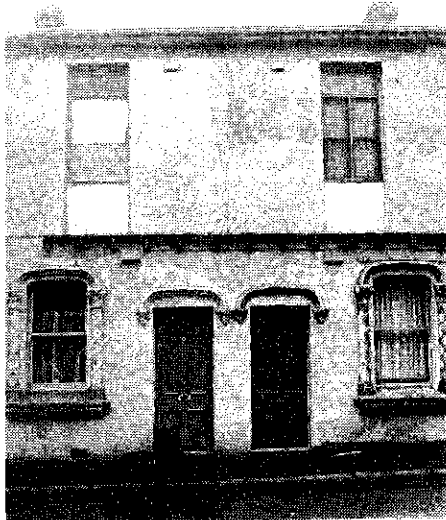
Poor Building Condition. Victorian detailing evident.
