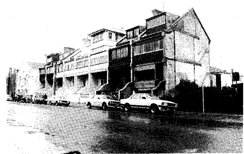
Unsympathetic Additions. Grott Ct. Low grade balcony enclosures. Attic extensions to front facade.
