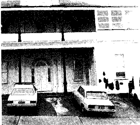
Former Sailor's Home - low quality unsympathetic additions.
