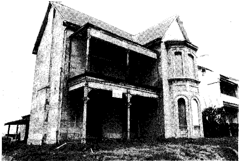
Former Station Masters House · Vacant · Poor Condition.
