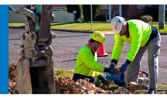
THIS WORK REDUCES THE RISK OF PIPE BREAKS AND HELPS MAINTAIN GOOD QUALITY DRINKING WATER Hunter Water is improving the water supply system by replacing aged and damaged watermains across our network. This work reduces the risk of pipe breaks and helps maintain good quality drinking water.
