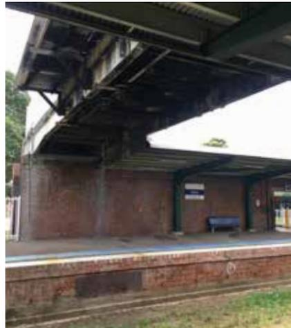
Figure 143: Underside of footbridge, showing steel structure
