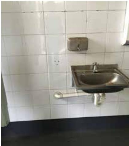
**Figure 134: Basin with drainage through wall to the ladies WCs**
