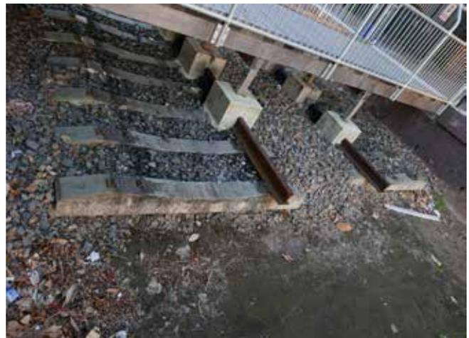
**Figure 79:** Footings of temporary bridge with remnant tracks and sleepers.
