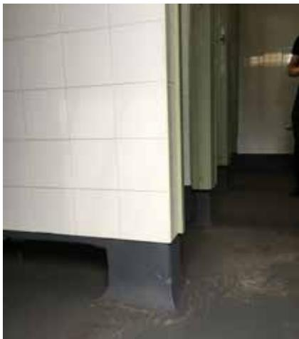
**Figure 137: Stall to floor junction**
