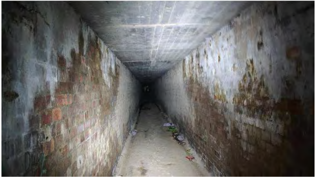
Figure 58: Internal view of the tunnel leading from the Searchlight Engine Room towards the Searchlight Bunker. Note the damp present to internal brick walls and the concrete roof. (Source: Duncan, Carol, "The Memorial Drive Tunnel," ABC Newcastle website, 20 August 2013, accessed 24 August 2017 via http://www.abc.net.au/local/photos/2013/08/20/3829654.htm )
