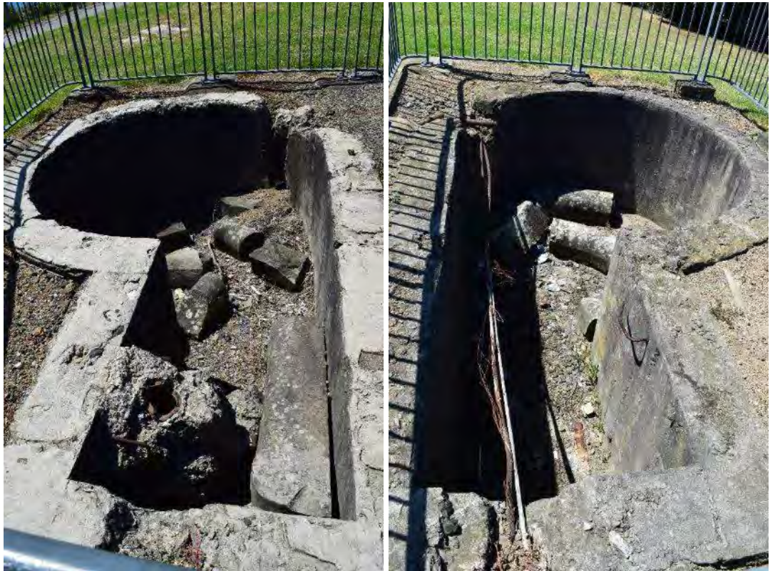
Figure 30: View of the DRF stations from above ground with the northern station pictured on the left and the southern station pictured on the right. These structures have been infilled with rubble present internally.
