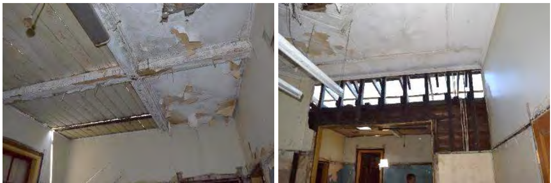
Figure 14: Weatherboard ceiling with crossed timber beams in a smaller ancillary room (left) evidence of decorative plaster moulding in the main living area (right). Note the damage incurred to the ceiling as a result of water ingress caused by openings to the roof following the April 2015 storm.
