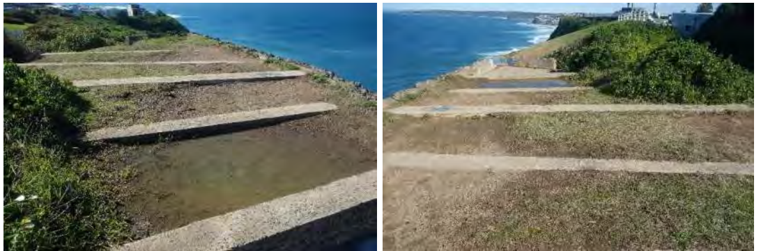
Figure 49: Views of the roof looking north east (left) and south west (right). Note the raised sections and vegetation present. This area also captures water as visible in the image on the right.
