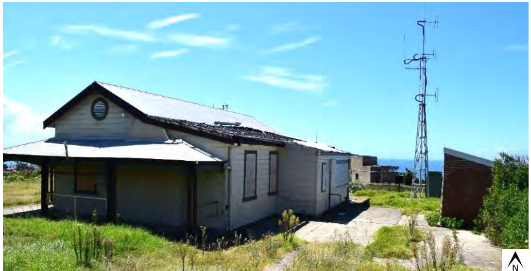
Figure 169: Image from 2016, showing the damage caused to the cottage following the storm of April 2015. The chimney was lost and damage was caused to the interiors.
