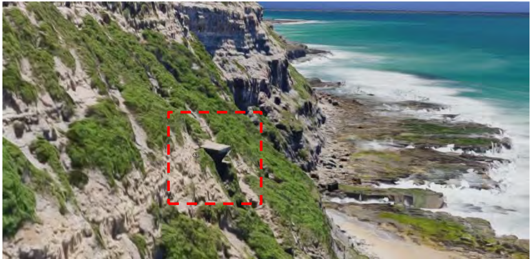
Figure 60: Oblique view looking north towards the southern elevation of the No.1 Searchlight. Note the structure recesses into the cliff face due to its size and the use of concrete. The design is similar to the Park Battery, no.1 gun and bunker. (Source: Google Maps 3D, accessed 30 August 2017 via https://www.google.com.au/maps/place/Strzelecki+Lookout/@-32.9388057,151.7759448,54a,35y,340.12h,79.25t/data=!3m1!1e3!4m5!3m4!1s0x6b73146c7dcb8503:0x771e4820b5c1be76!8m2!3d-32.9368196!4d151.7770135 )
