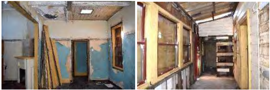
Figure 19: Internal views of the Dining Room where picture rails and skirting have been removed (left) and the former bathroom, located in Sunroom 2 (right, southern extension).
