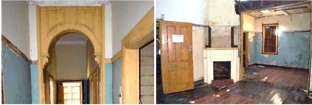
Figure 13: Entry hallway with decorative timber architraves and corbels (left) remaining fireplace and timber floors (right). The masonry fireplace was installed in the 1920s and was substantially damaged in the April 2015 storm. It is also leaning into the room and is not considered to be in a typical style from the 1920s.
