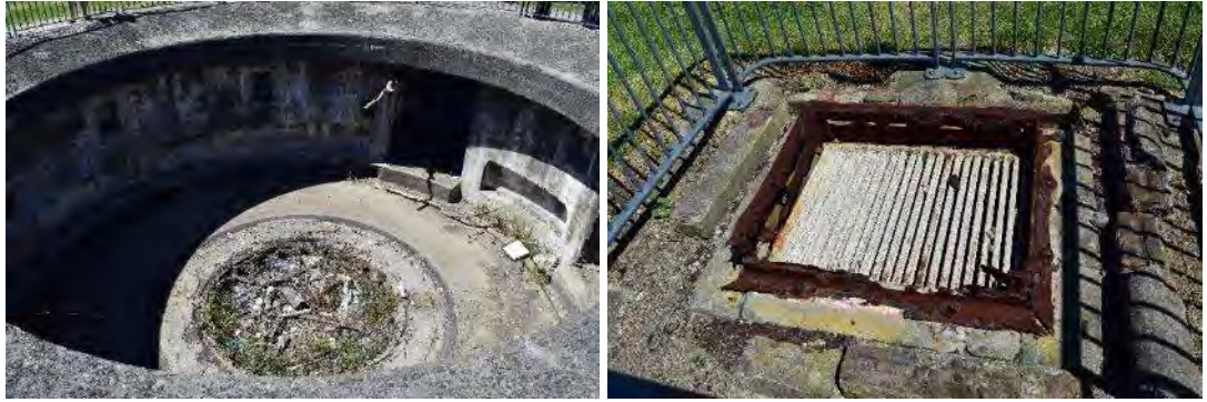
Figure 29: Views of the gun pit and skylight/vent from above ground. Note the corrosion to the skylight and rubbish present within the gun pit. The gun pit is also partially shaded by the concrete edge.
