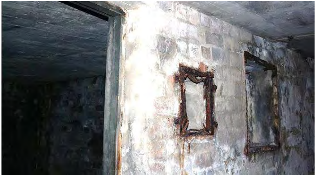
Figure 59: Another view within the tunnel leading to the Searchlight Bunker. Corroded metal framing is visible around openings. (Source: Duncan, Carol, "The Memorial Drive Tunnel," ABC Newcastle website, 20 August 2013, accessed 24 August 2017 via http://www.abc.net.au/local/photos/2013/08/20/3829654.htm )
