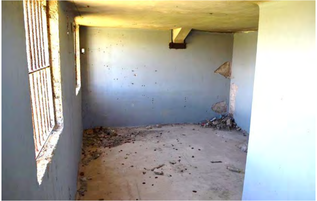
Figure 41: Internal view of Room 2, located on level 3. Evidence of paint finishes can be seen and damage to interiors. This room is in a better condition to some of the other rooms within the Battery Observation post.
