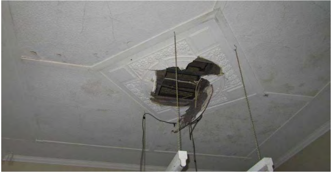
Figure 252: Photograph of the ceiling of the living room showing the damage caused by the storm. (Source: photographs taken by John Carr and provided by Newcastle City Council)
