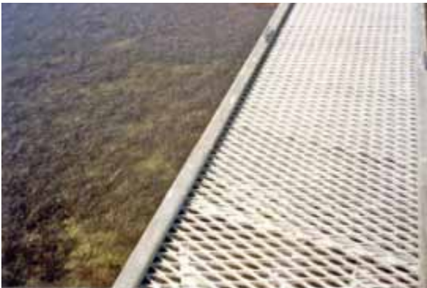
Figure 10. Mesh decking can be used to reduce the impacts of shading on seagrasses.
