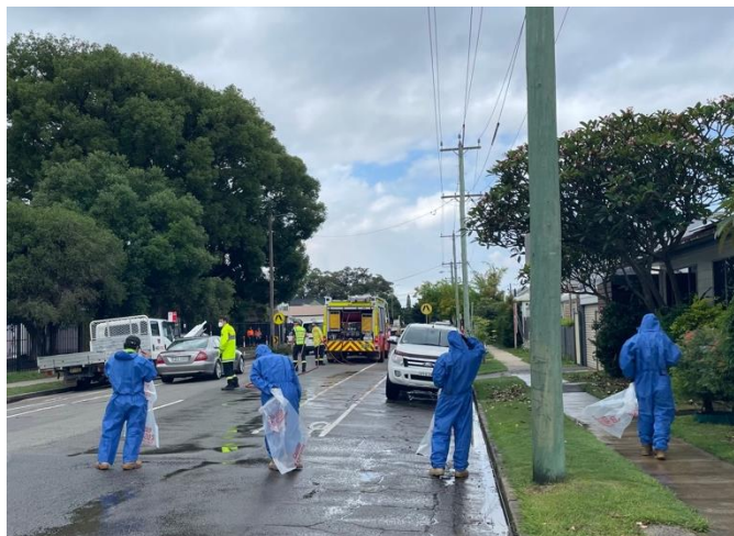
Specialist asbestos contractors cleaning up an impacted street.
