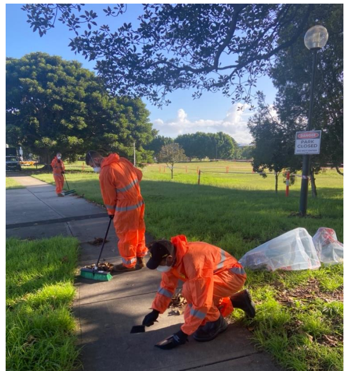
Specialist asbestos contractor cleaning at Islington Park.
