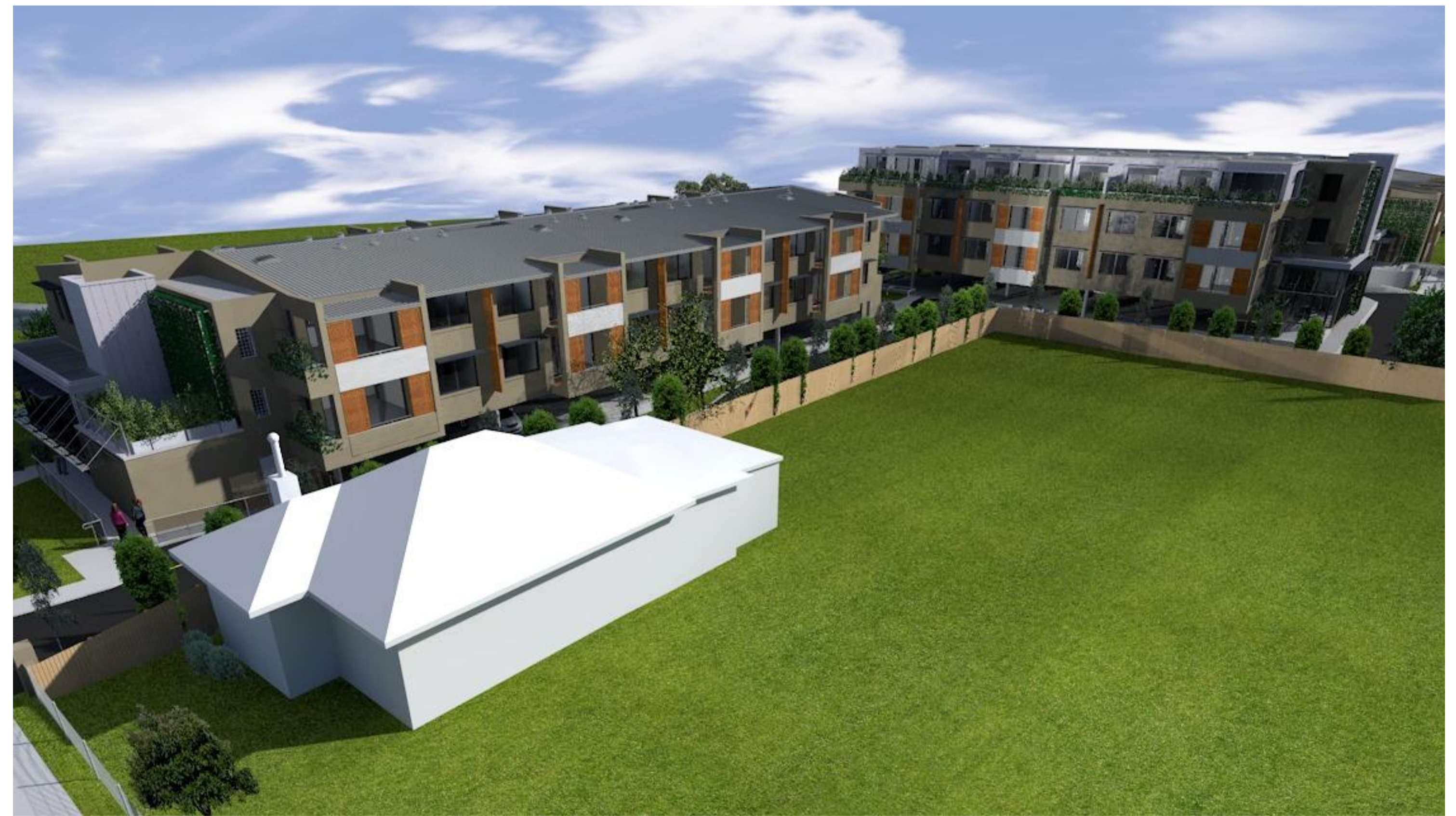
4 Aerial View from Northeast
