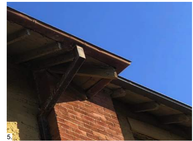
FURTHERMORE, THE EAVES LINING BOARDS ARE DIFFERENT ACROSS THIS SECTION OF ROOF
