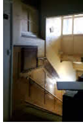
6 STAIRCASE TO FIRST FLOOR NON-ORIGINAL FABRIC. BRASS HANDRAIL c1930s RETAINED FOR REUSE IN PROPOSED LOBBY
