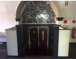
7 ORIGINAL ENTRY WAY LOOKING FROM 1875 COX BUILDING TOWARD LATER ADDITIONS. ORIGINAL BLAUSTRADE MAY BE CONCEALED WITHIN PLASTERBOARD NIB WALLS
