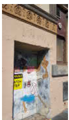
15 FIRE EGRESS CUT THROUGH EXISTING EXTERNAL WALL ALONG SCOTT STREET, ALTERED ORIGINAL WINDOWS
