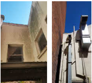
14 NON-ORIGINAL GLAZING FACING LIGHTWELL. NOTE MULTIPLE SERVICES CONNECTING TO/THROUGH THIS ZONE.
