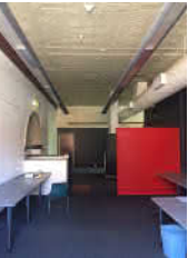
10 FULL HEIGHT PARTITION INTERSECTS ORIGINAL CEILING. FULL HEIGHT RISER AND AC DUCT ALSO PENETRATE CEILING.
