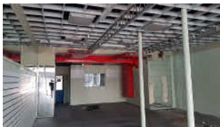
11 SIGNIFICANT ALTERATION TO INTERNAL FABRIC INCLUDING FALSE CEILINGS AND POORLY INTEGRATED SERVICES
