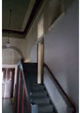
12 MODIFIED OPENINGS AND NON-ORIGINAL STAIR TO CREATE CONNECTION BETWEEN CHANGE IN FLOOR LEVELS
