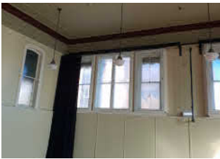
1 ORIGINAL GLAZING WITH ADDITIONAL MODERN UNIT FIXED TO INSIDE FACE. ORIGINAL LIGHTING FIXTURES PRESENT WITHIN FORMER LIBRARY SPACE.
