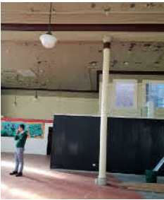
2 ORIGINAL STEEL COLUMN EXPOSED IN FORMER LIBRARY SPACE, SUPPORTING EXPOSED BEAM.
