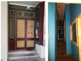
5 ENTRY DOORS TO SERVICE CORRIDOR AND FIRST FLOOR. BELIEVED TO BE PERIOD APPROPRIATE, MODIFIED AND REPURPOSED FROM ELSEWHERE IN THE BUILDING - MAY BE REUSED
