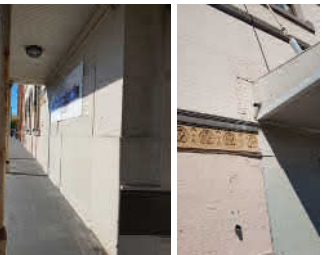
1 INFILLED FORMER OPENING IN EXISTING BRICKWORK VISIBLE. PAINTED-OVER FEATURE TILING AND FOUNDATION PLAQUE TO SHOPFRONT APPARENT.
