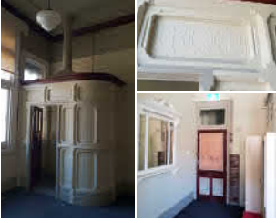
5 ORNATE WC AND EXPOSED LATH AND PLASTER ADJACENT MODERN LIFT.
