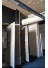
9 FULL HEIGHT PARTITIONS INTERSECT ORIGINAL CEILINGS. ELECTRICAL/ COMMS/AC THROUGH THIS ZONE, INCLUDING FULL HEIGHT MECH RISER.
