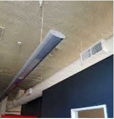
8 EXISTING PRESSED METAL CEILINGS GENERALLY GOOD CONDITION, RETAIN FOR REINSTATEMENT
