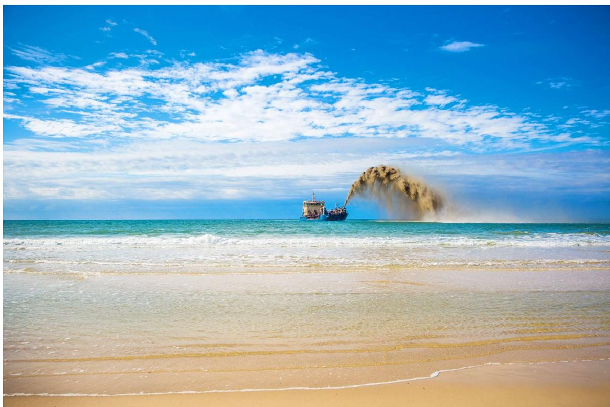
Figure 4: A TSHD rainbowing sand onto the nearshore area of the beach as part of beach nourishment works (source: City of Gold Coast).
