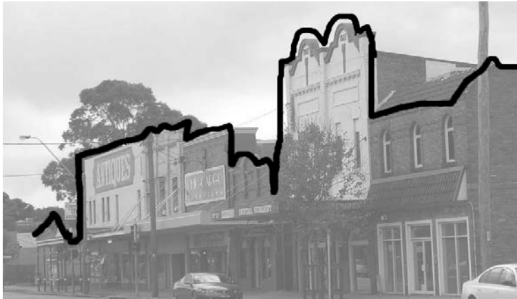
Figure 6: Existing parapets dominating the street edge
