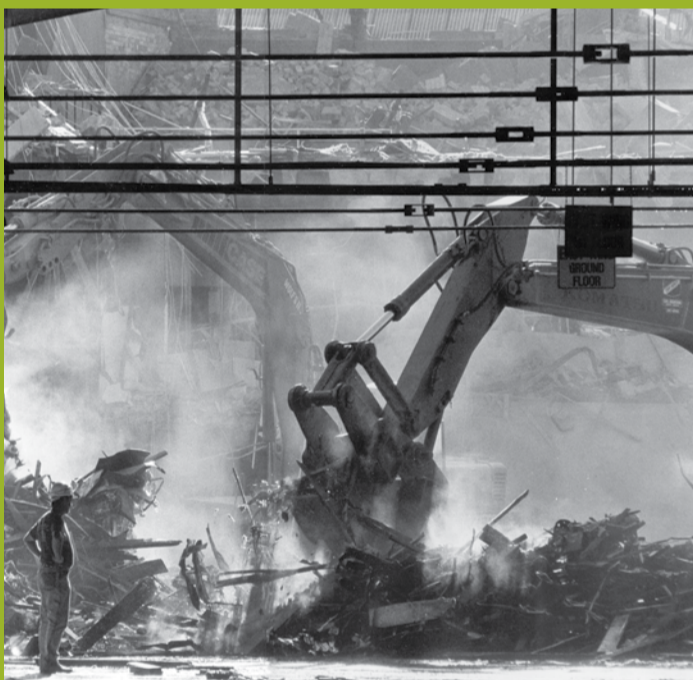
Demolition of the Worker Club, December 1989
